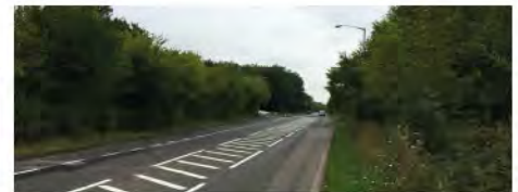
View 7. North Dane Way
