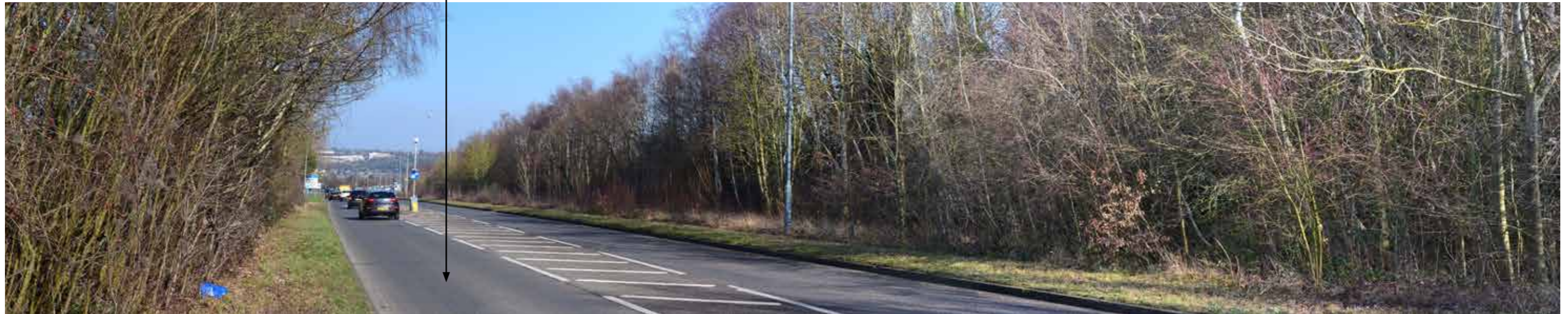
VIEW 3: North Dane Way south of Shawstead Road at Whites Wood, Wayfield, Chatham
