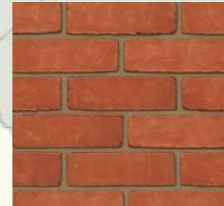
Red colour brick walls
