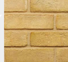
Buff colour brick walls
