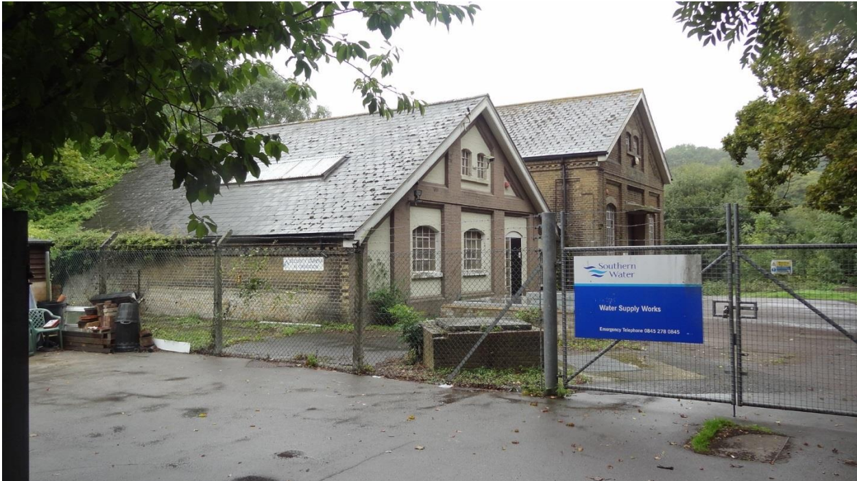
Figure 11 – Southern Water pumping station south of Capstone Road roundabout
