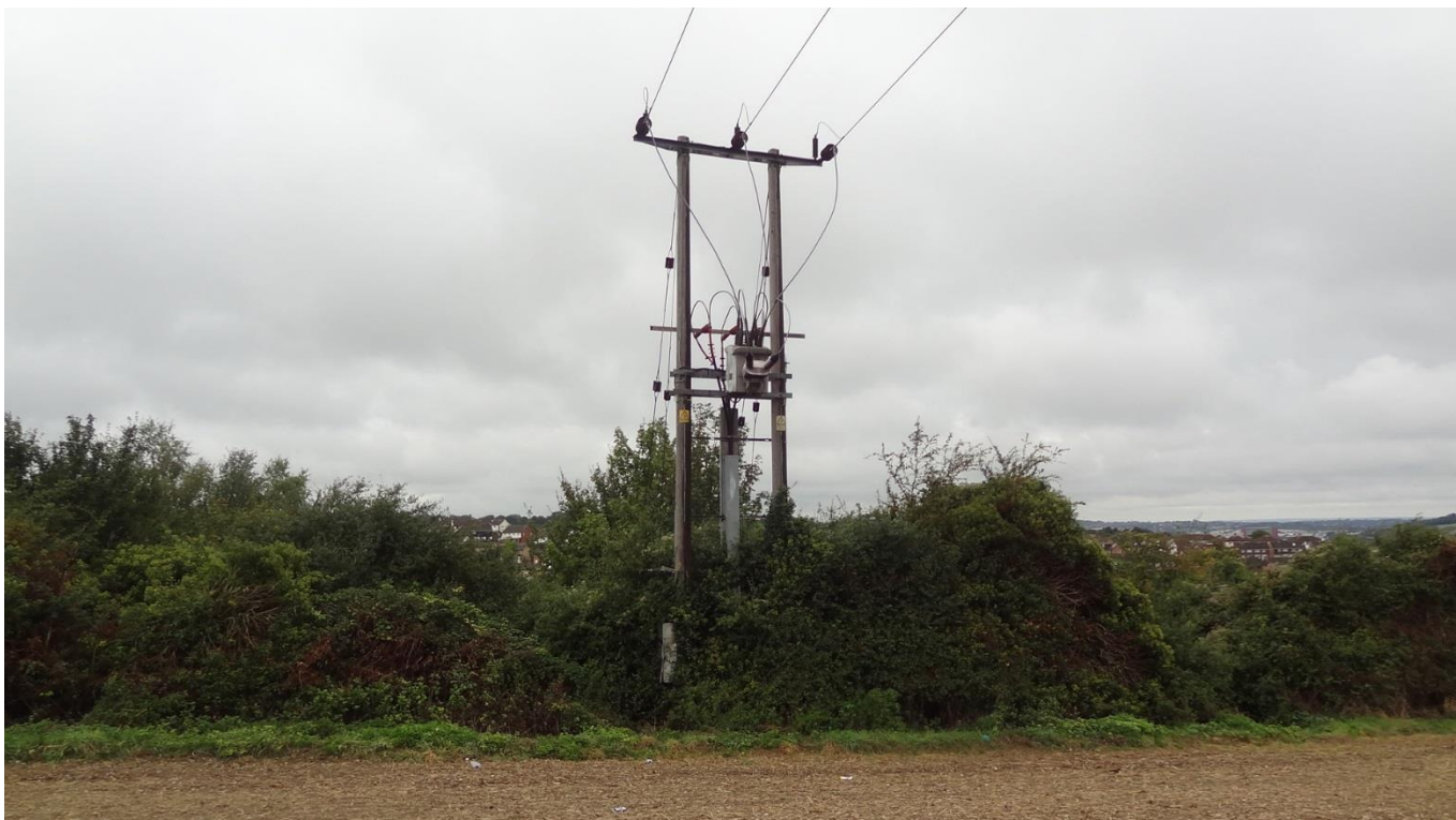
Figure 3 – North Dane Way GVR in northwestern area of the site
