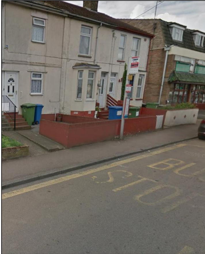
Figure 2.6 – Minster Road Westbound Bus Stop
