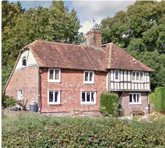
Asymmetric composition, hipped and half-hipped roofs, hanging clay tile detail, jettied upper storey with timber detail
