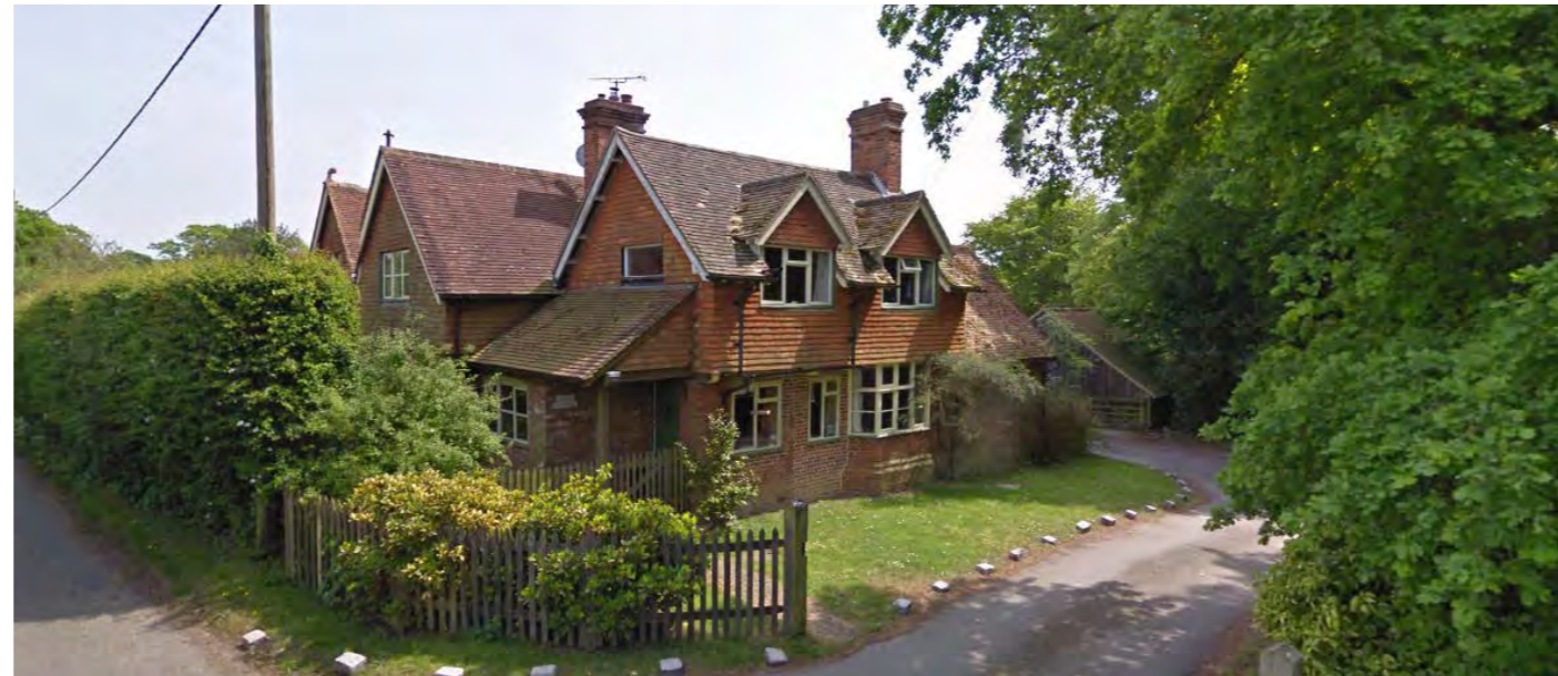
Upper storey clay tile hanging, mixture of window types, asymmetric brick chimneys
