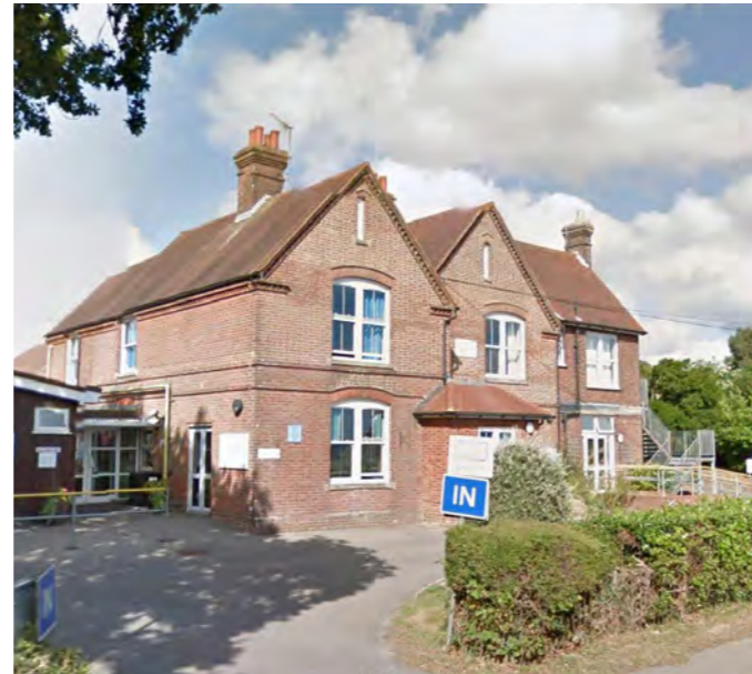
Well detailed brick gable with verge detail, brick arches and string courses, combination of projections and setbacks that break up massing
