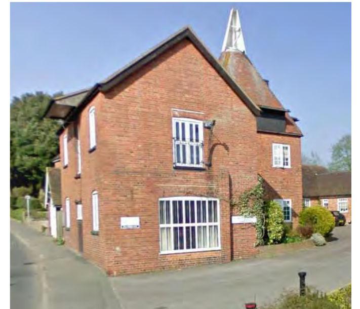
Symmetrical brick gable, varying window types, black painted timber barge-boards, strong urban frontage to street
