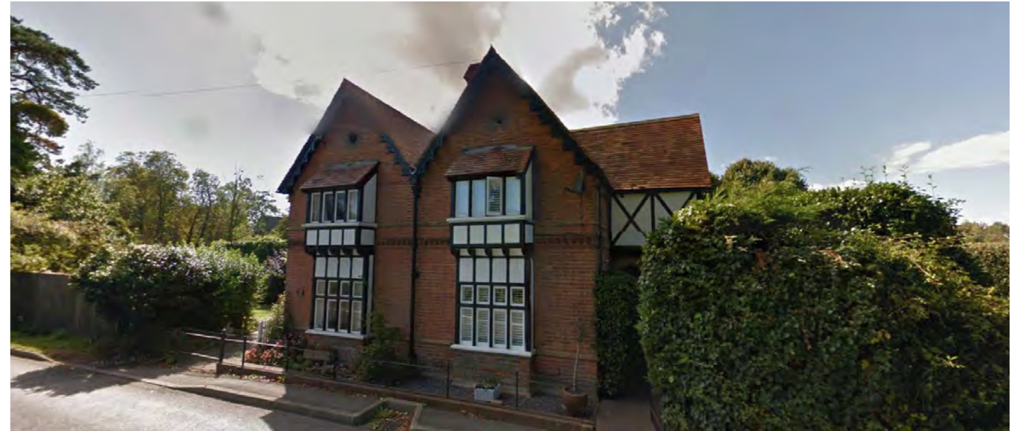
Paired brick gables with painted timber barge-boards
