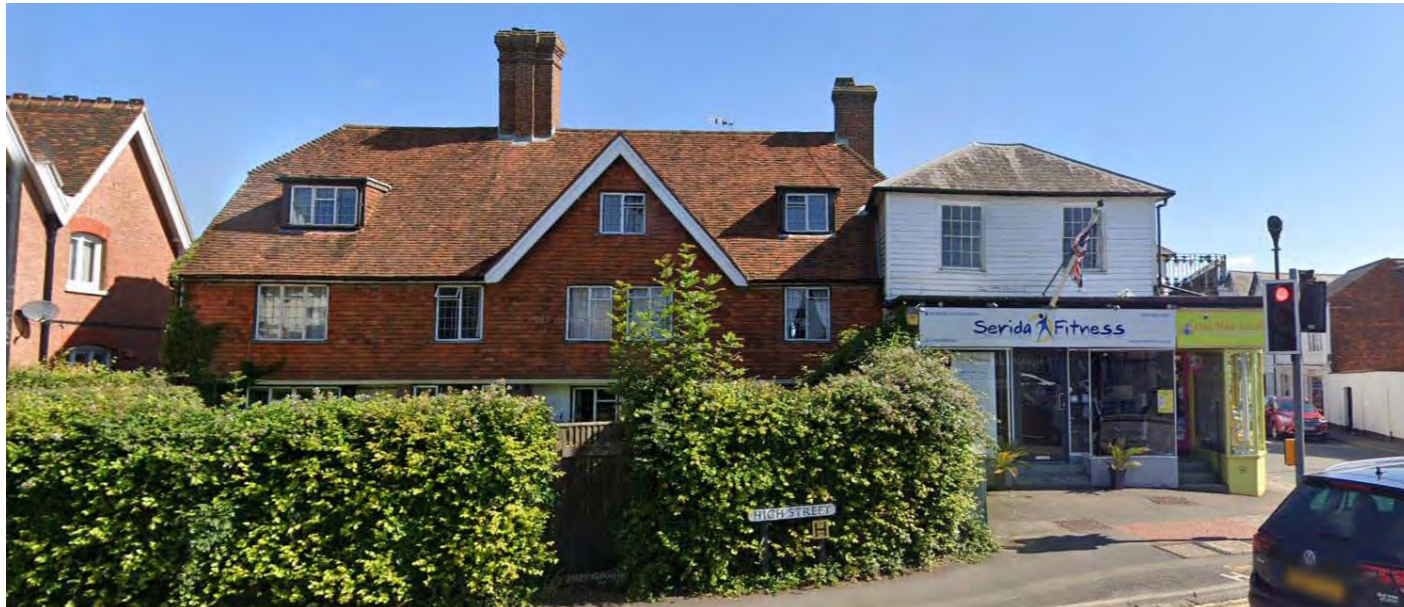
Asymmetric composition, projecting hanging clay tile gable with timber barge-boards, mixed cladding materials at different heights
