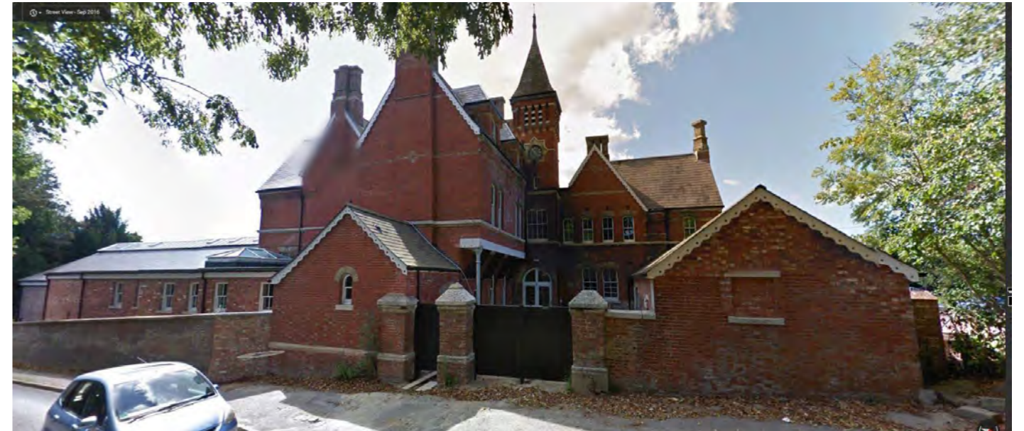
Brick detailing, decorative timber barge-boards, contrasting use of gables, chimneys and overall massing creates visual interest
