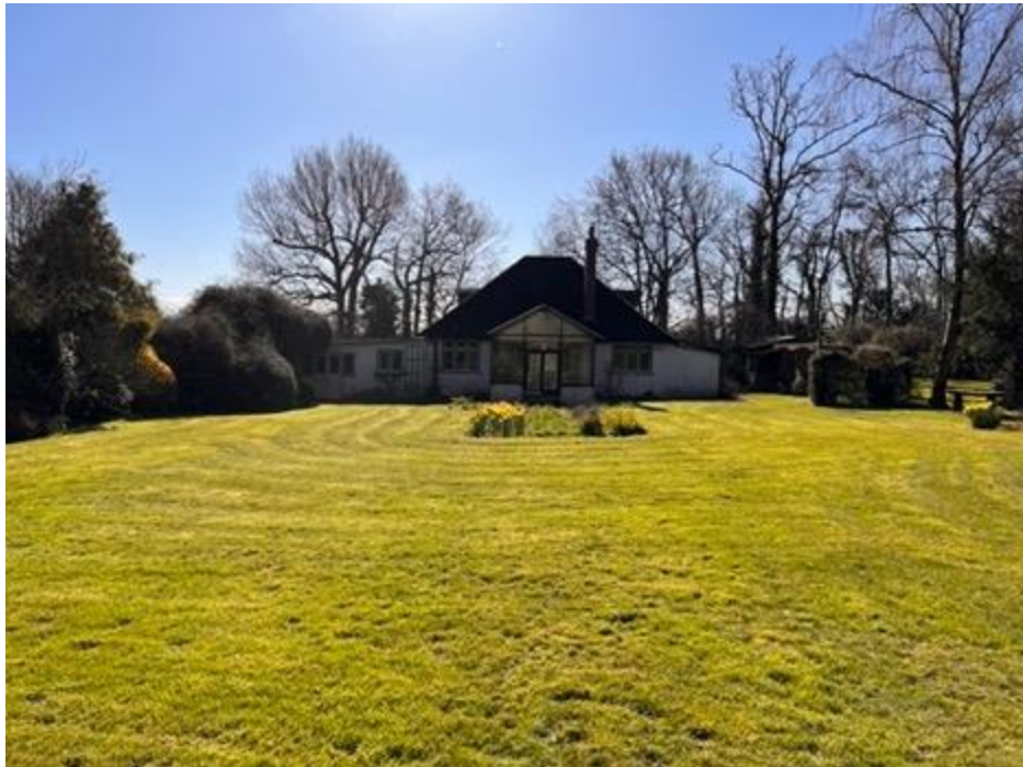
View of rear elevation of Russetings from the rear garden
