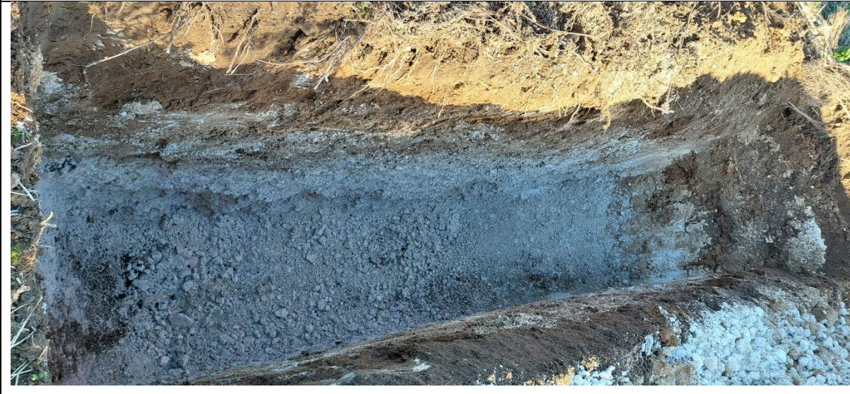
TP24 – Finished trial pit
