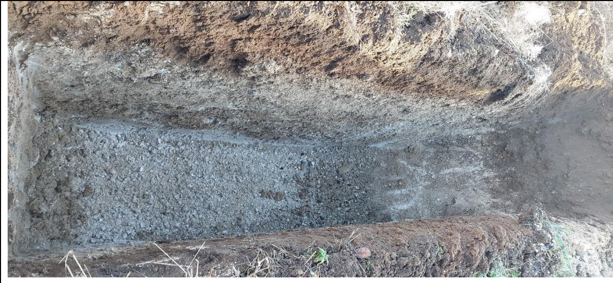
TP32 - Finished trial pit
