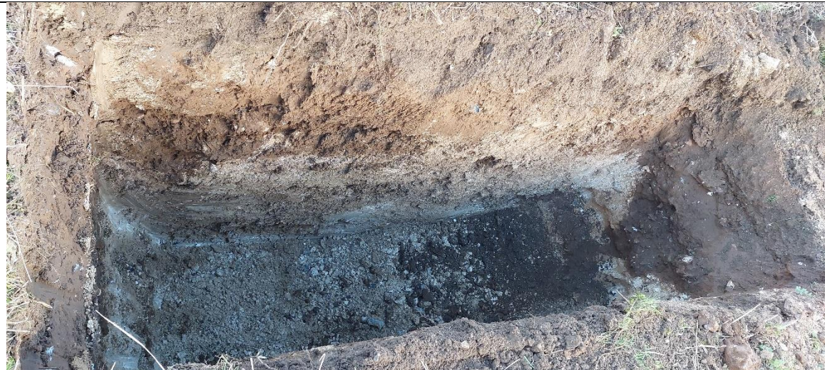
TP35 – Finished trial pit
