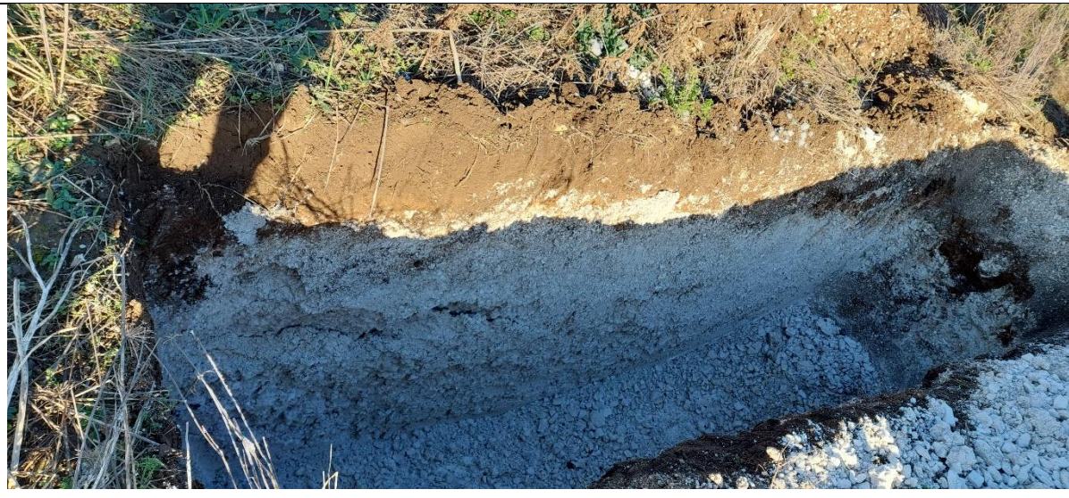
TP25 - Finished trial pit
