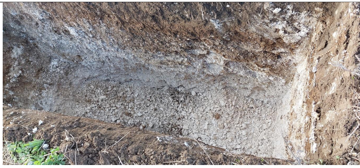
TP33 – Finished trial pit
