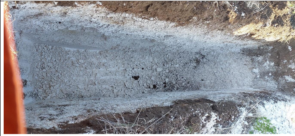
TP30 - Finished trial pit
