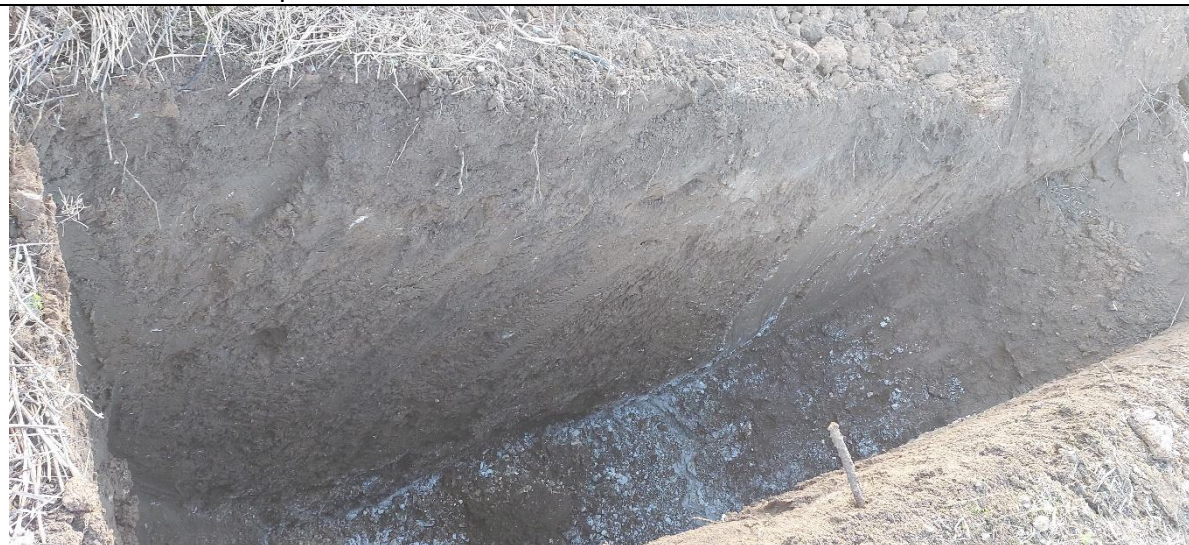
TP20 – Finished trial pit
