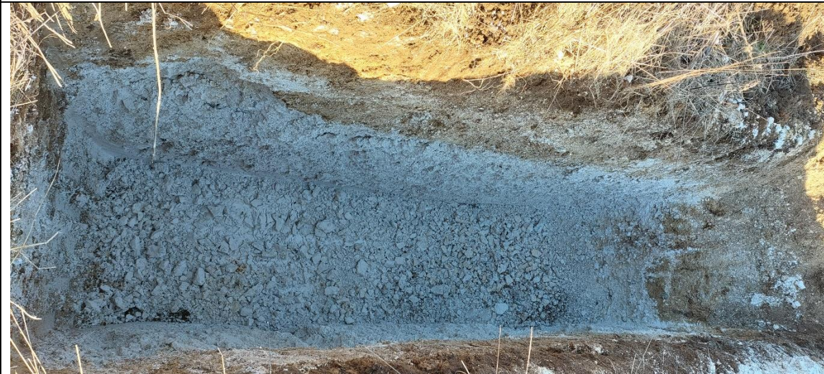
TP14 – Finished trial pit
