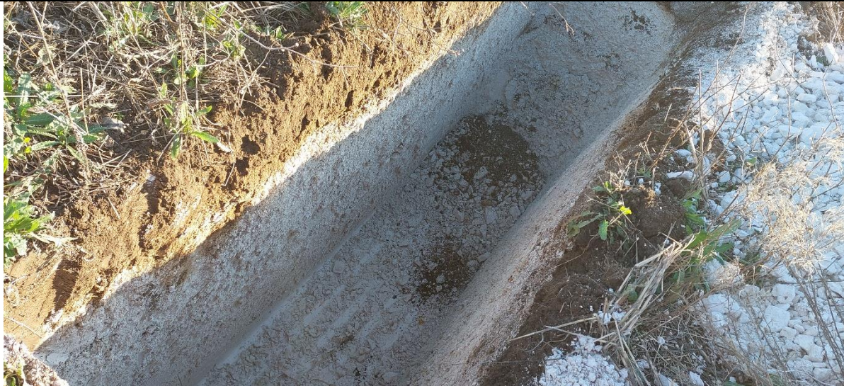
TP22 – Finished trial pit
