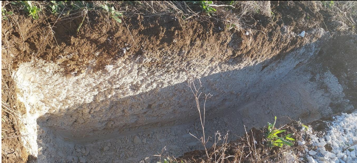
TP16 – Finished trial pit
