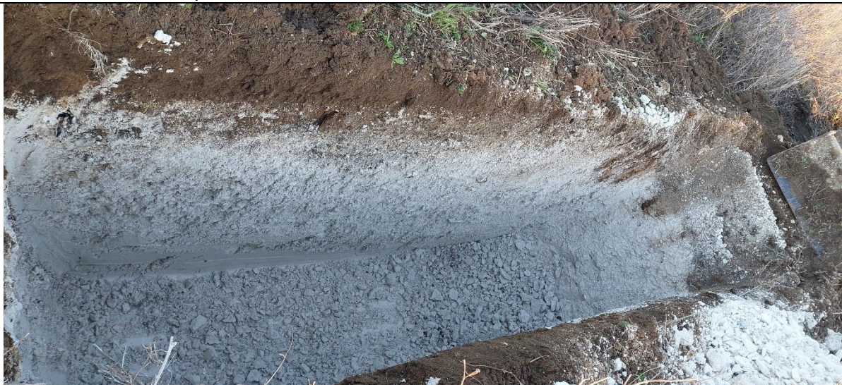
TP21 – Finished trial pit
