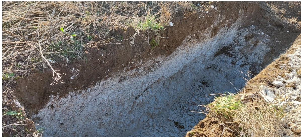
TP27 – Finished trial pit
