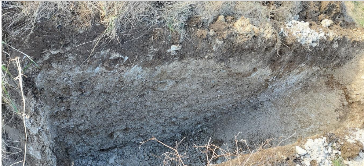
TP19 – Finished trial pit
