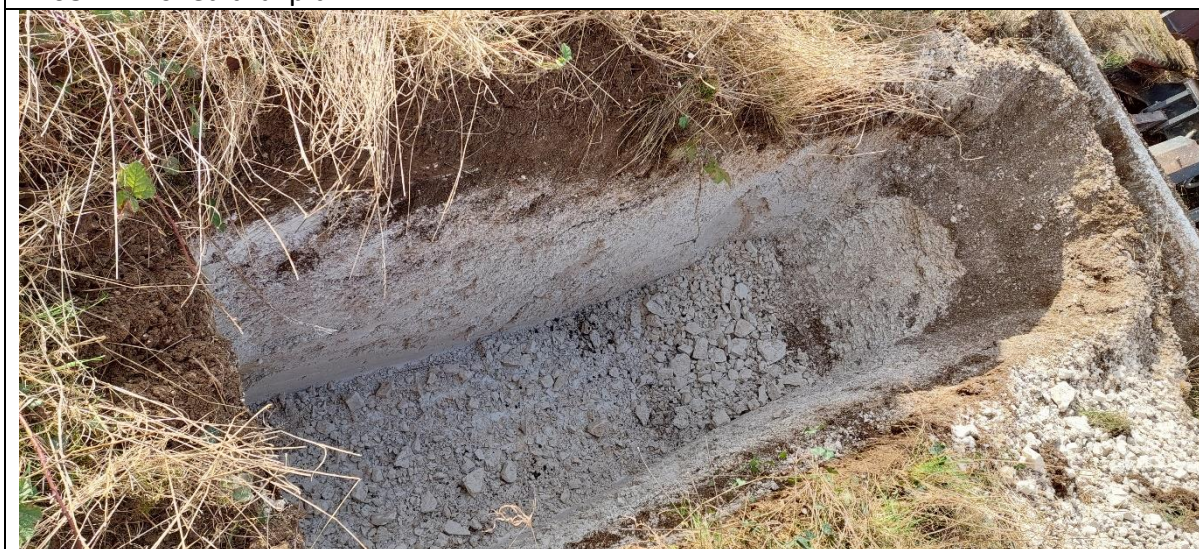
TP08 – Finished trial pit
