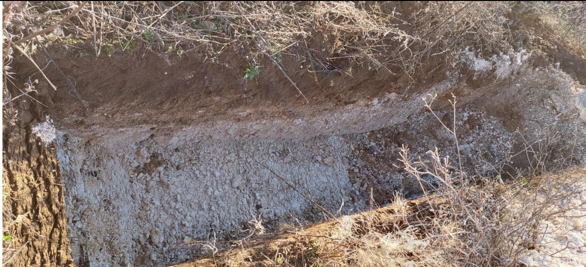
TPA – Finished trial pit
