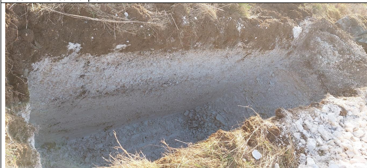
TP03 – Finished trial pit
