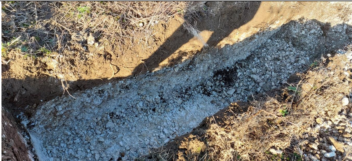
TPB – Finished trial pit
