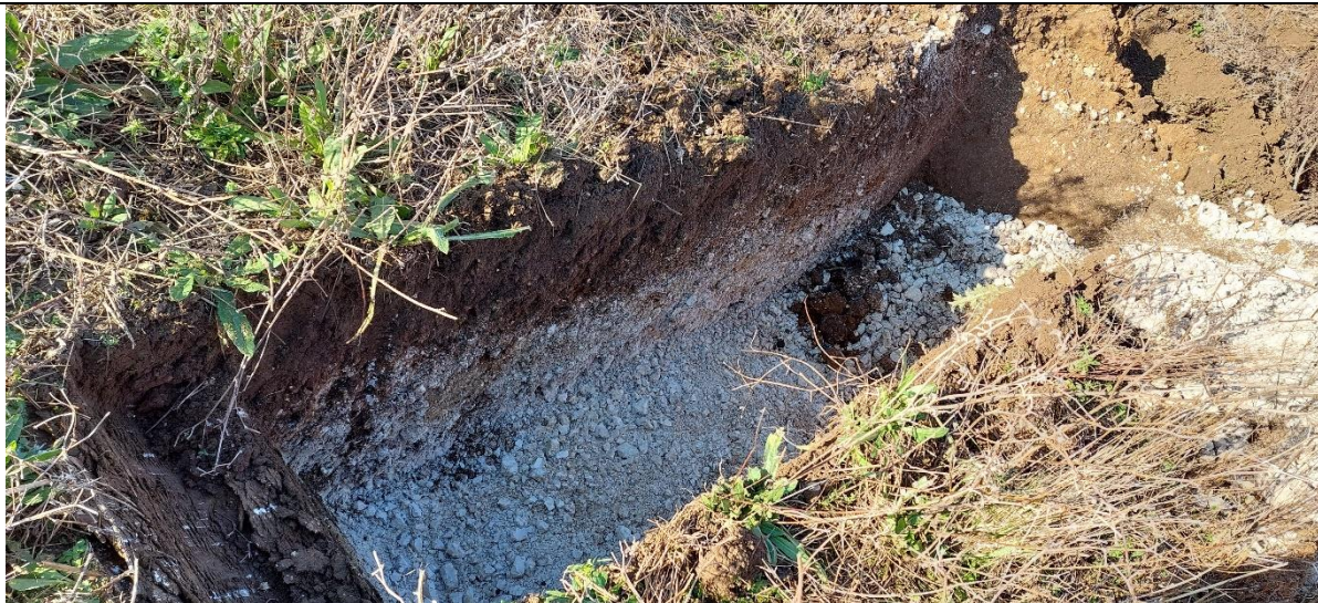
TPC – Finished trial pit
