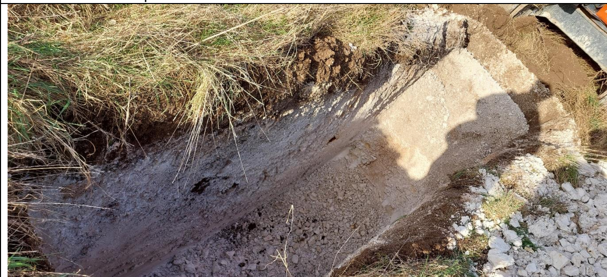
TP07 – Finished trial pit
