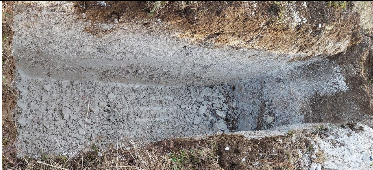
TP06 – Finished trial pit
