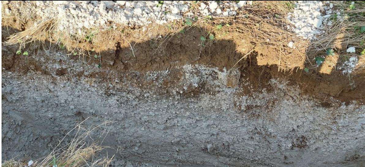
TP04 – Finished trial pit
