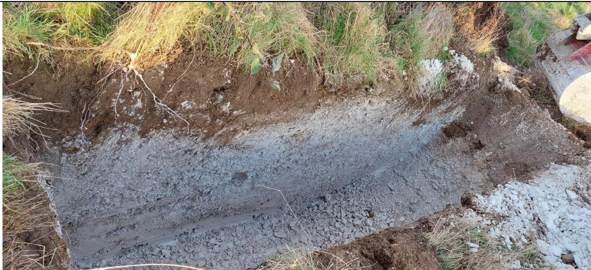
TP02 – Finished trial pit
