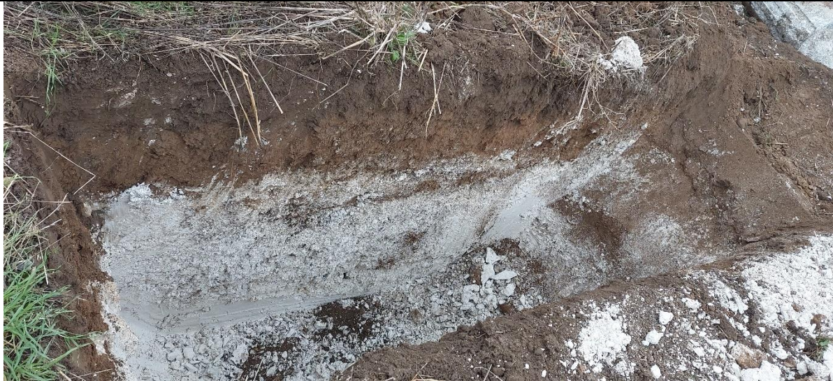
TP13 – Finished trial pit
