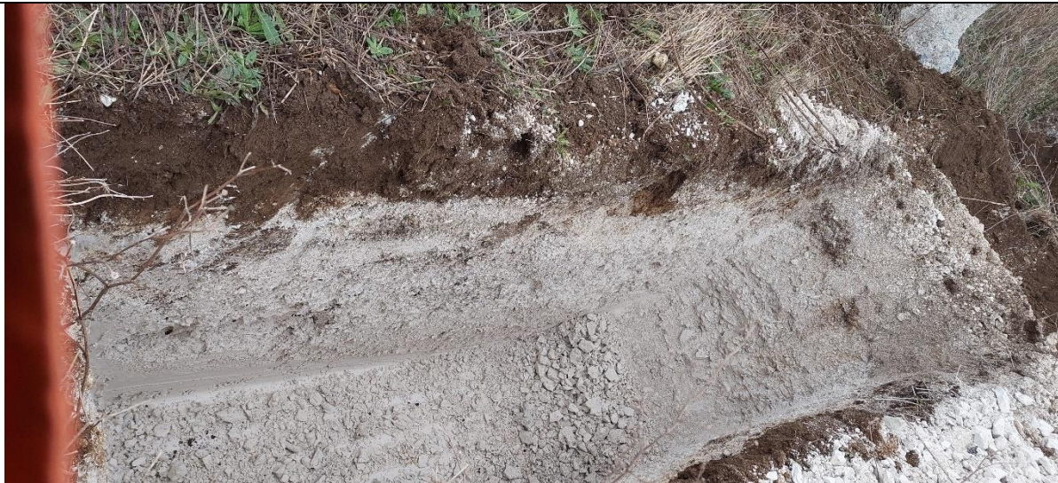
TP12 – Finished trial pit
