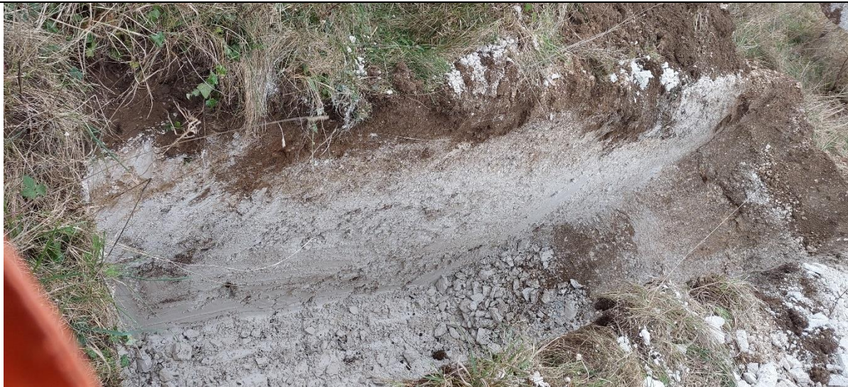
TP10 – Finished trial pit
