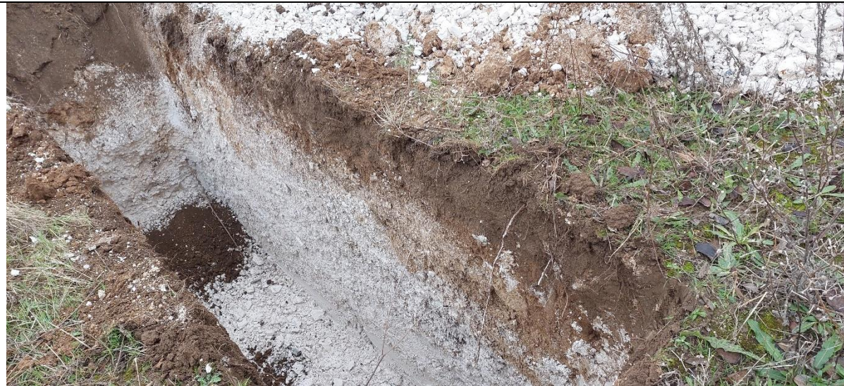
TP11 – Finished trial pit
