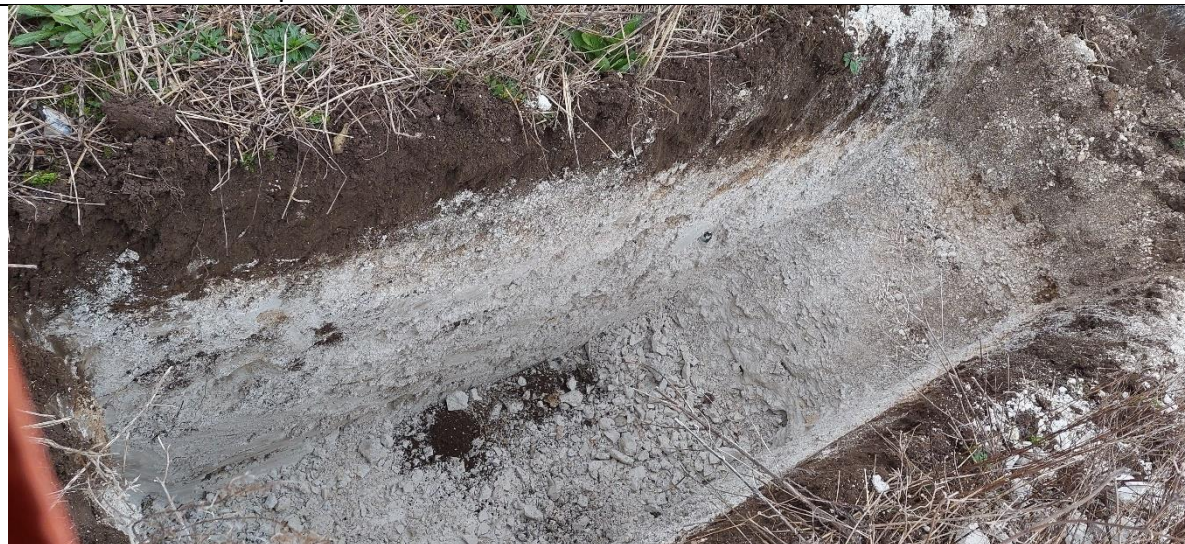
TP17 – Finished trial pit
