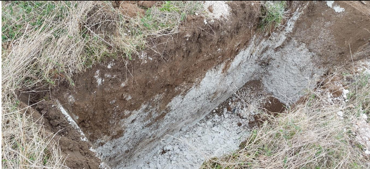
TP09 – Finished trial pit
