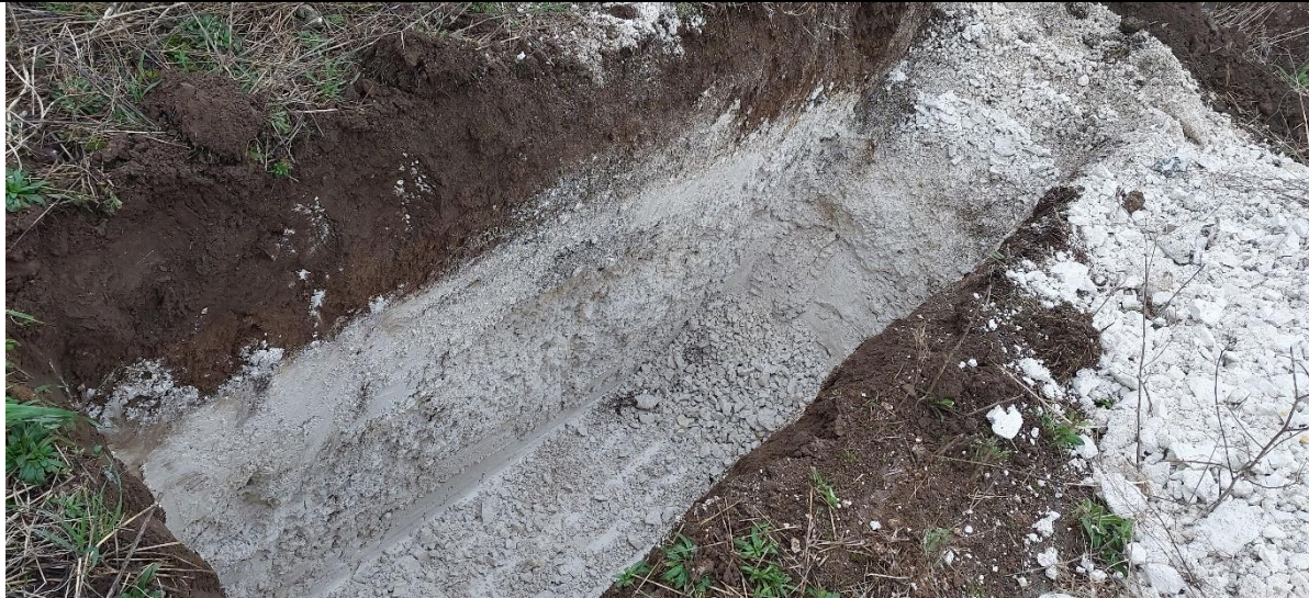
TP18 – Finished trial pit
