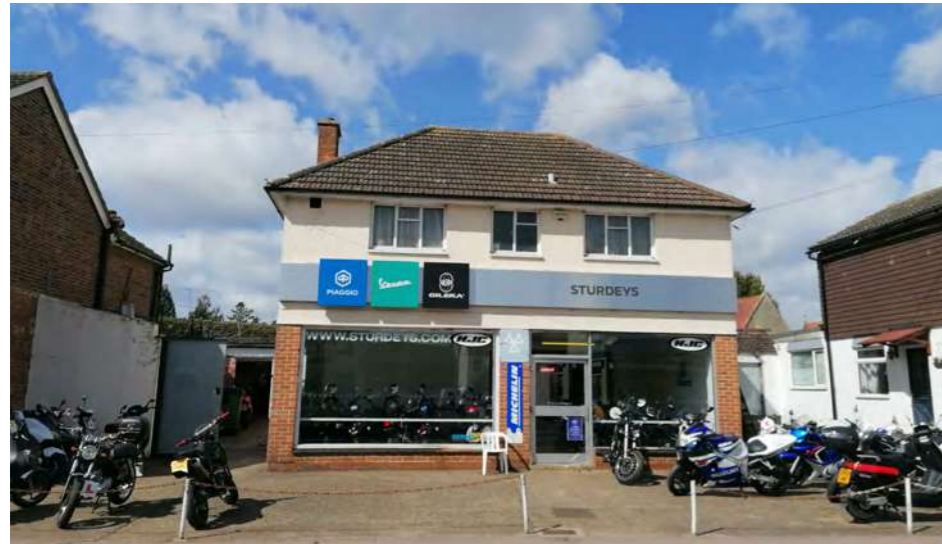
1. FACING WEST TOWARDS THE EXISTING GARAGE PRIMARY ELEVATION
