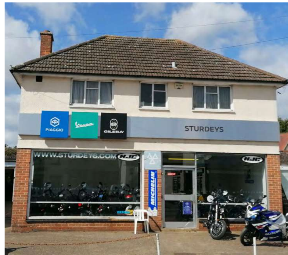
THE EXISTING BUILDING (PRIMARY FACADE)
