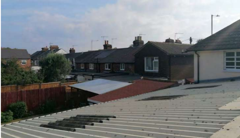
5. FACING N.EAST TOWARDS THE REAR ELEVATIONS OF NO. 96
