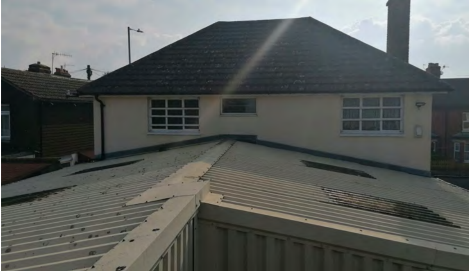
4. FACING EAST TOWARDS THE REAR ELEVATION OF THE 2-STOREY UNIT
