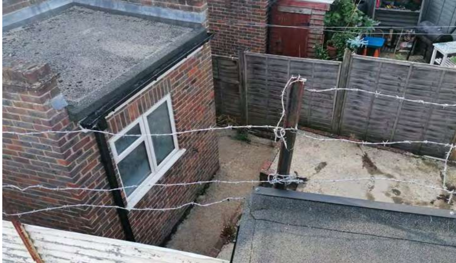
3. FACING SOUTH TOWARDS REAR AMENITY SPACE OF NO.94
