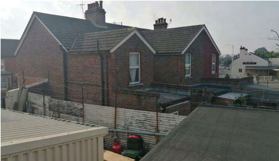
7. FACING S.EAST TOWARDS THE REAR ELEVATION OF NO. 94
