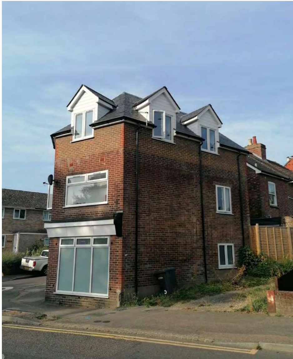
1. ADDITIONAL STOREY ADDED TO EXISTING CORNER SITE
