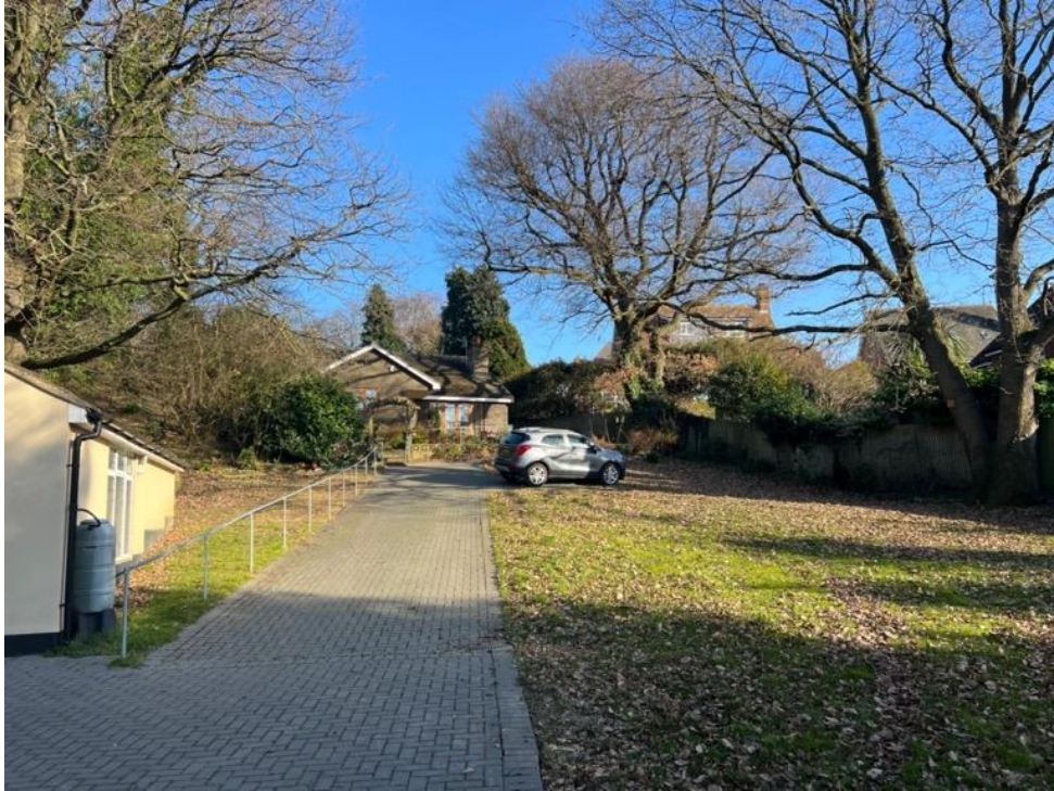
View 1- front elevation of Greenwood Lodge from the driveway, with garage just visible in the foreground
