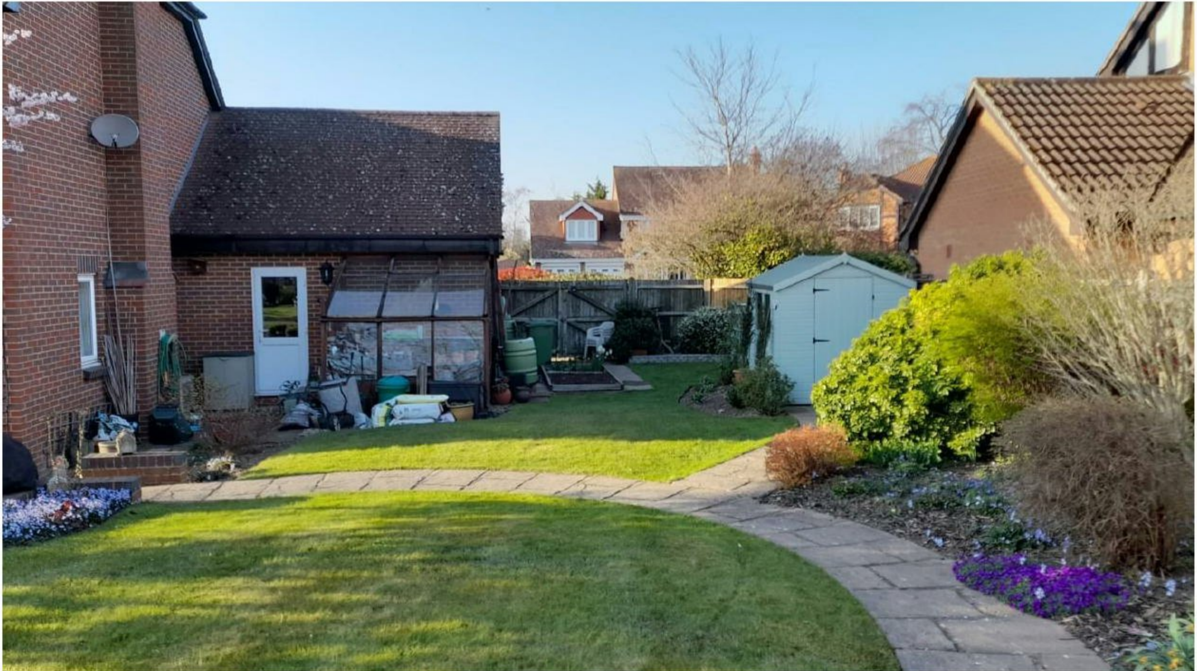
The Site viewed from the South
