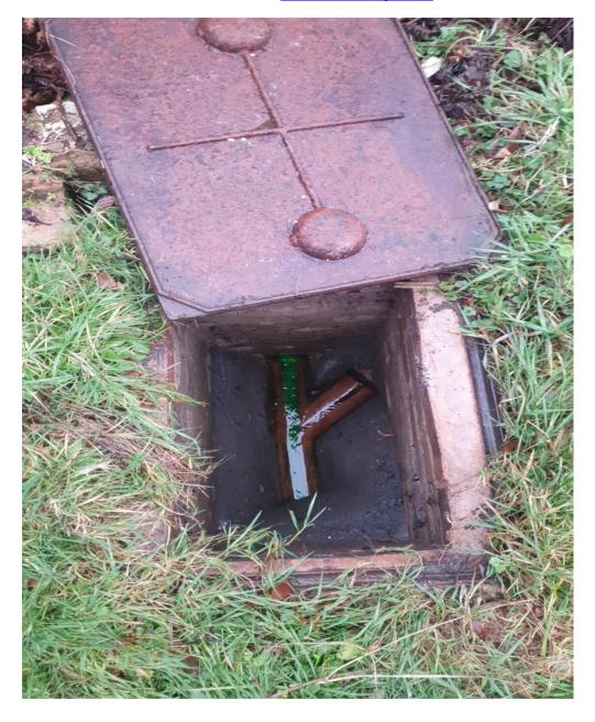
In Photo Above this is Manhole 2 showing the green tracing dye which was used in the Rain water gulley flowing into the foul system.
