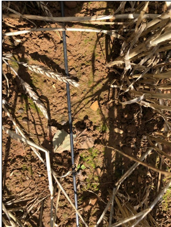
Plate 9. Black cable identified on northern perimeter of Site boundary.
