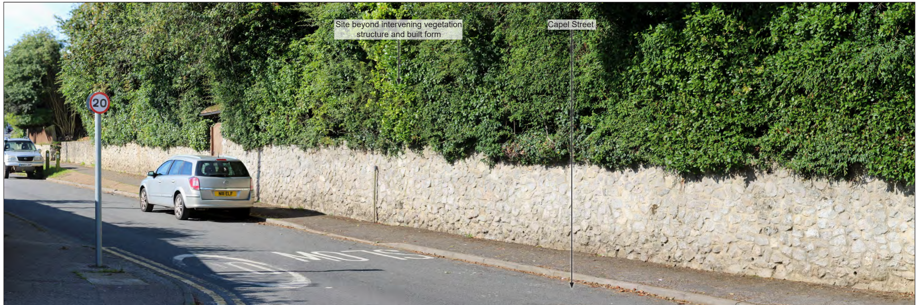
Viewpoint Coordinates: E 624860, N 138719 Date & time of photograph: 16/08/2023 09:12 AOD & Viewing height: c. 153m AOD 1.6m Weather conditions: Clear, good visibility. Viewpoint 1 (Annotated Panorama Image for Context Only)
