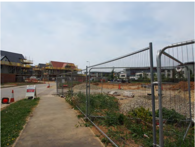
New development on former airfield at Hawkinge
