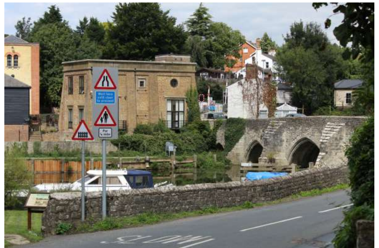
Photograph 4 – East Farleigh Bridge
