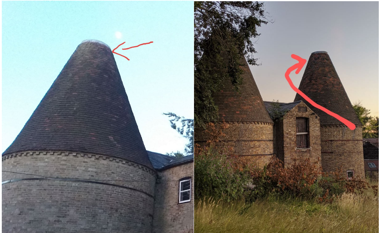
Figure 3: surveyors' photos indicating roost access point for common pipistrelle in B1 oast roundel
