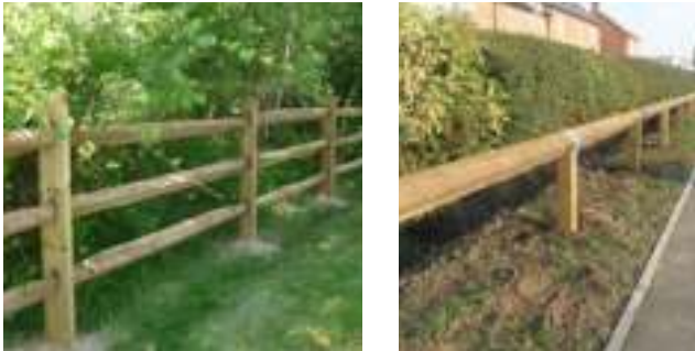
Timber post and rail/ knee rail fencing to enhance the rural/ urban fringe character of housing development
