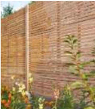
Contemporary timber fencing to divide private gardens. Combined with amenity planting where fencing fronts on to the streetscape
