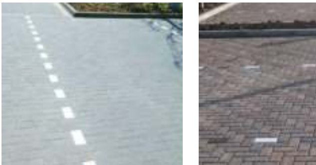
Block paving marker blocks provide subtle delineation between the pedestrian and vehicle areas, promoting a relaxed shared surface space.
