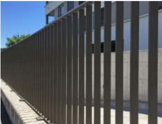
Contemporary railings compliment the natural stone vernacular of the proposed feature walls
