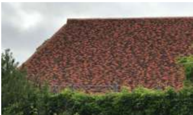
Manor Farm Barn roof
