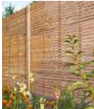
Contemporary timber fencing to divide private gardens. Combined with amenity planting where fencing fronts on to streetscape
