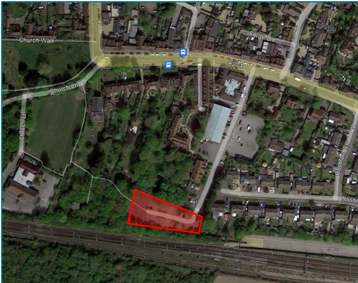
Figure 3.1 - Aerial View of the Existing Site
