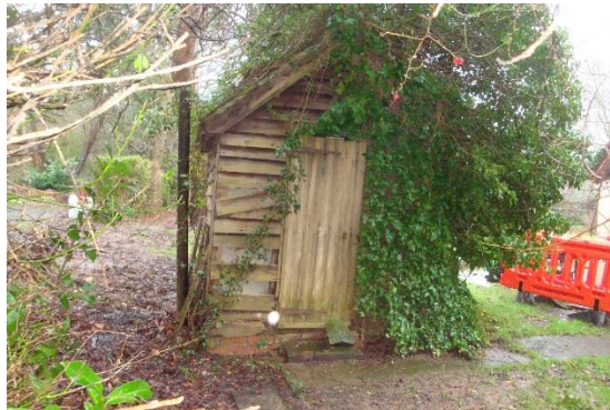
Existing outside WC
